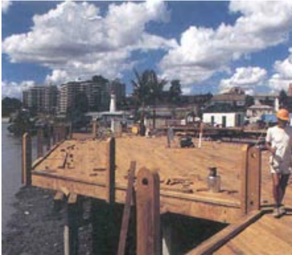
High traffic areas, such as the Expo '88 Boardwalk, require appropriate species selection and structural design to provide good serviceable life.
