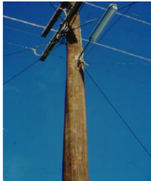
PEC-treated utility pole. (Photo courtesy Dr. Harry Greaves)
