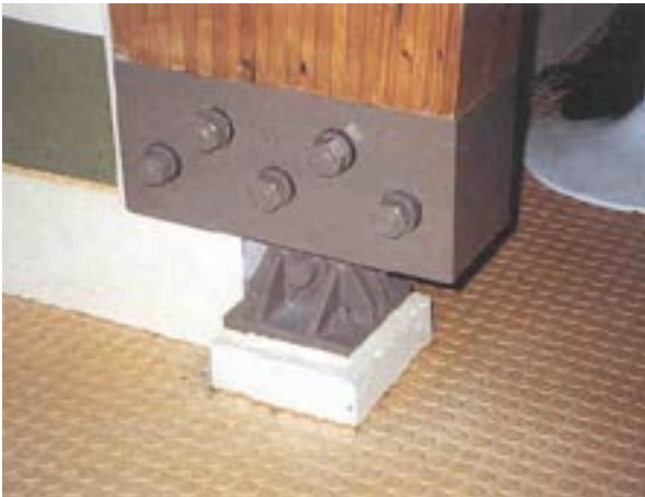
Stainless steel base connection and spacing block keeps timber columns clear of wet floor area.
