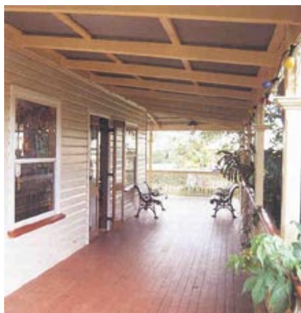
Traditional veranda provides shelter and protection to timber cladding and decking.
