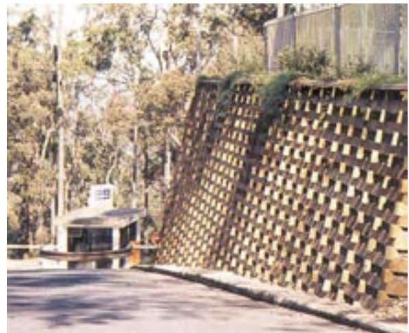
Durable hardwood (sapwood preservative treated) in a crib retaining wall.
