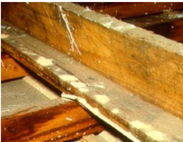
Lyctus borer produces a fine powdery frass when it attacks the starch-containing sapwood of hardwood roof timbers.
