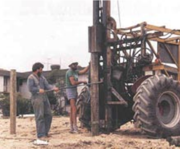
Preservative treated piles must be suitable for hazard level 5.
